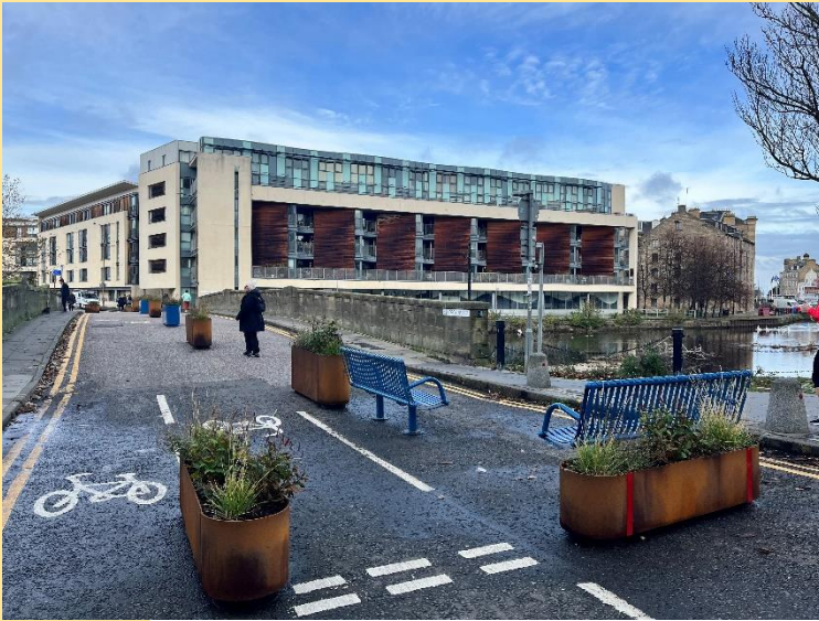
Street planters in Leith
